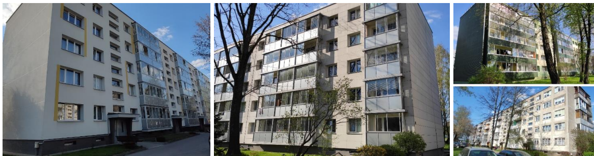
Fig. 11. Renovated and non-renovated buildings. Photographs by Anastasiia Kiuppier 11 pav. Renovuoti ir nerenovuoti pastatai. Anastasiia Kiuppier nuotraukos
