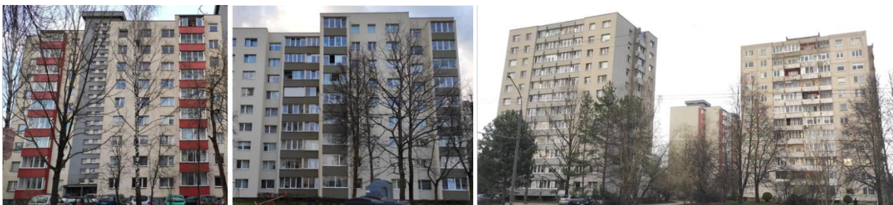
Fig. 4. Renovated and non-renovated buildings in the analyzed area. Photographs by Anastasiia Kiuppier 4 pav. Renovuoti ir nerenovuoti pastatai analizuojamoje teritorijoje. Anastasiia Kiuppier nuotraukos
