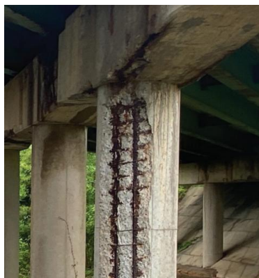
Fig. 2. Reinforcement corrosion of a bridge column (American Society of Civil Engineers, 2025)
